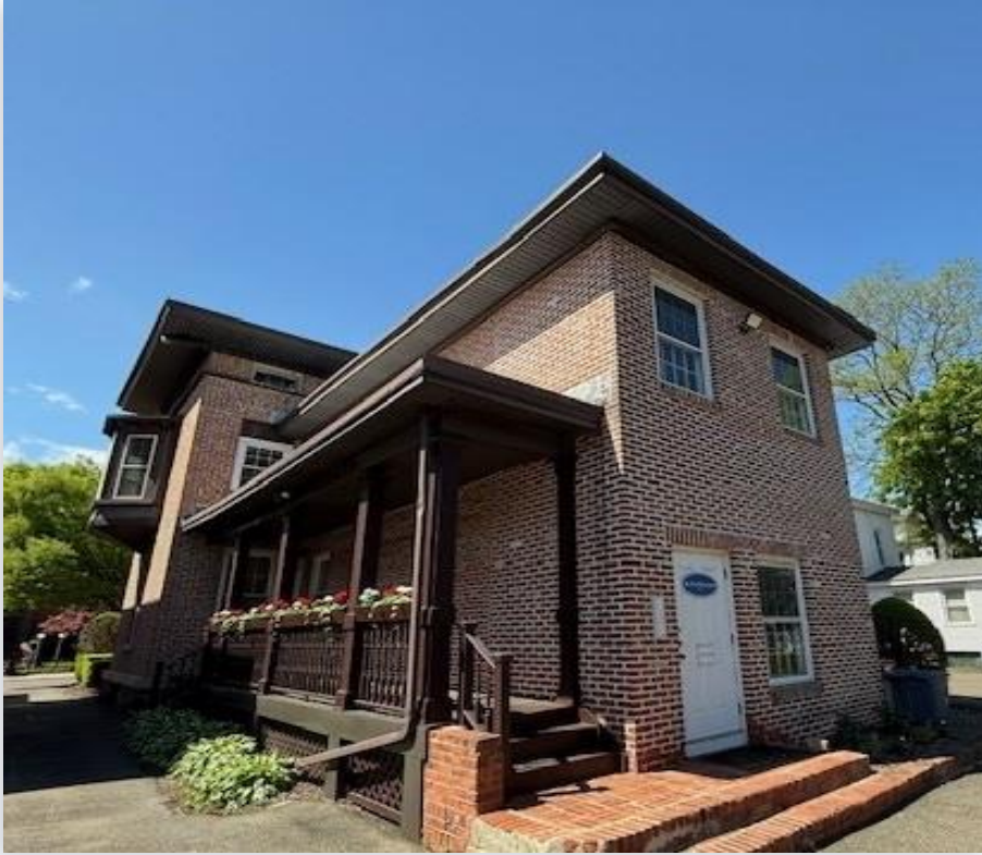
Side view & driveway — access to rear parking lot
